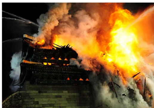
Figure 7: Fire in Sungnyemun
